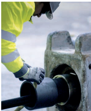
Insert the new bushing
