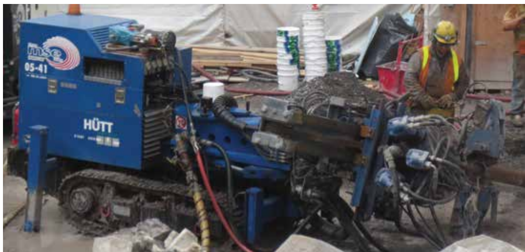
When headroom isn't a factor, severe angles can be. Some of the TAM bores were drilled under walls at 6 degrees from horizontal.
