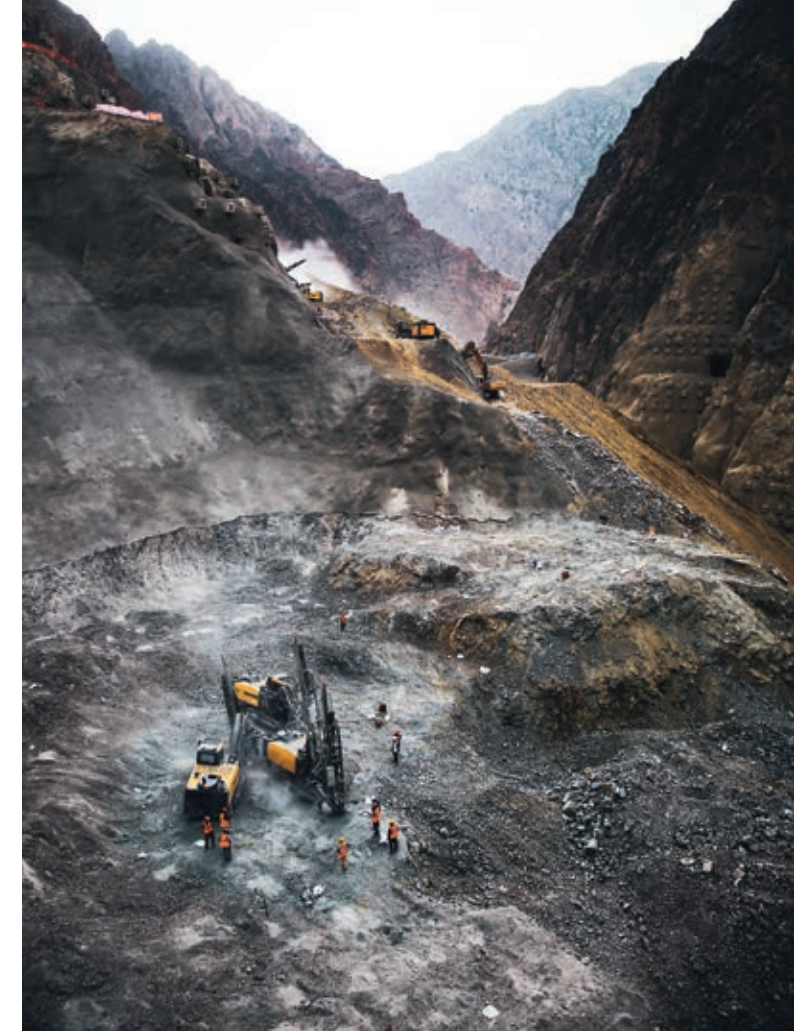
The dam body in what will be the Yusufeli Dam is being lowered by 275 meters. SmartROCT40 rigs are the key to success.
