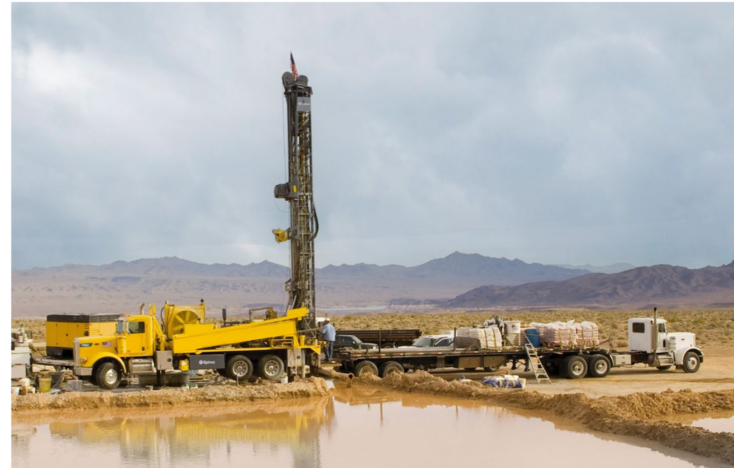
Blasthole drilling machine.
